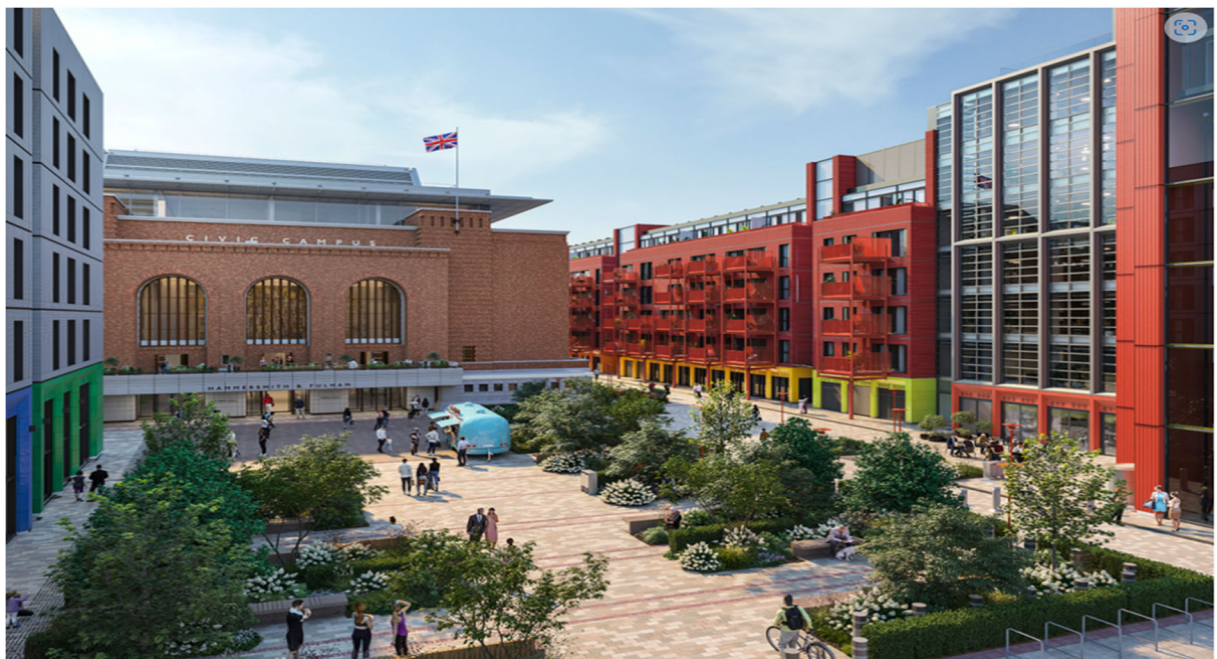
Figure 8: new homes and offices at the Civic Campus
